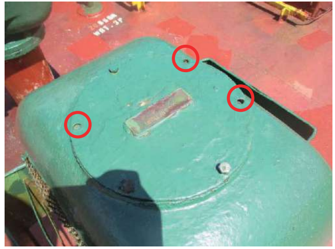
Missing bolts of air pipe head
