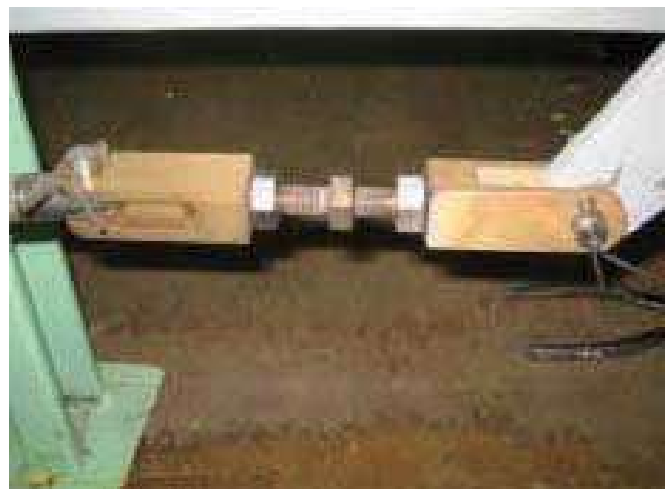
Correct condition of turn buckle
