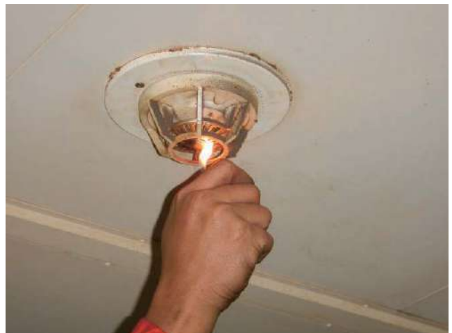
Inadequate test method
