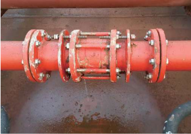
Leakage of fire line
