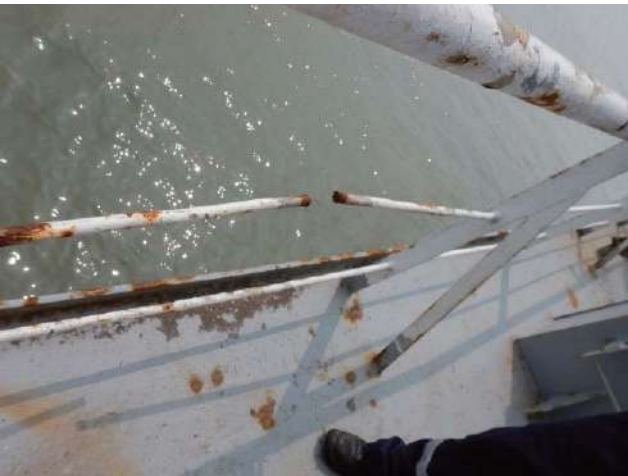
Damaged handrails
