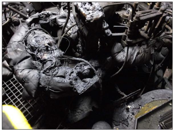
Figure 5b: Fire damage to burner unit
