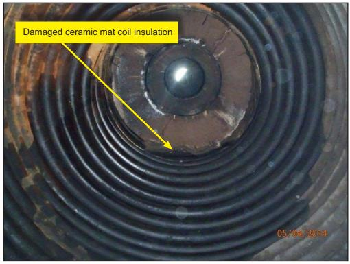
Figure 12: Photograph of internal view of port thermal oil heater furnace roof showing burner unit aperture and damaged insulation
