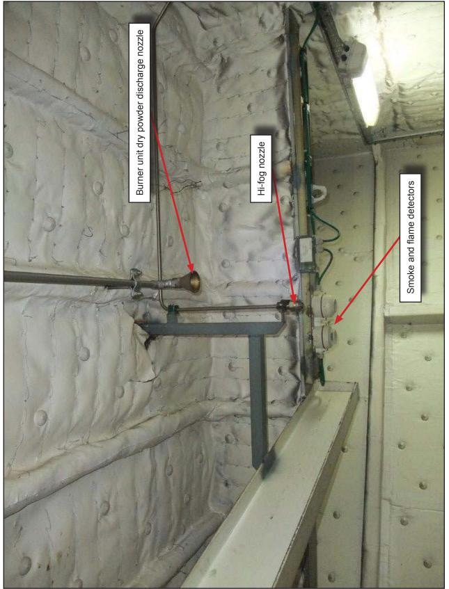
Figure 8: Photograph of boiler room fixed fire-extinguishing systems
