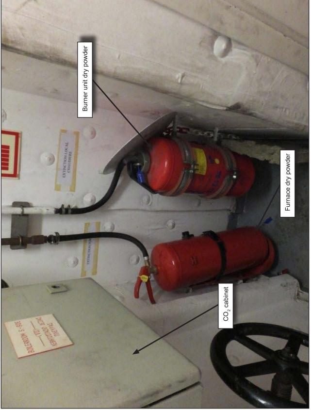
Figure 9: Photograph of fixed fire-extinguishing system control position
