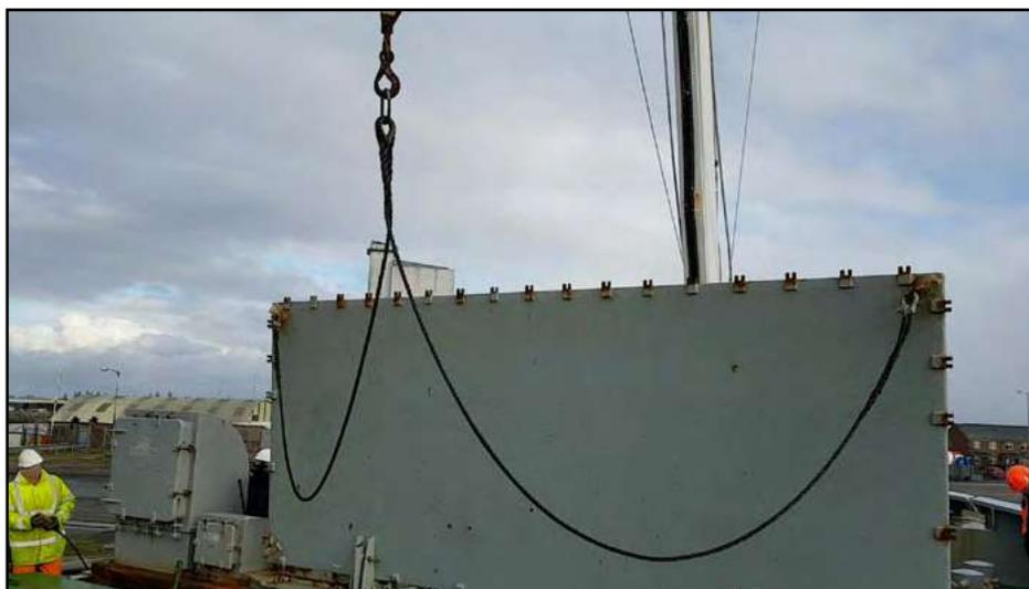
**Figure 4:** Hatch cover slings attached to crane hook
